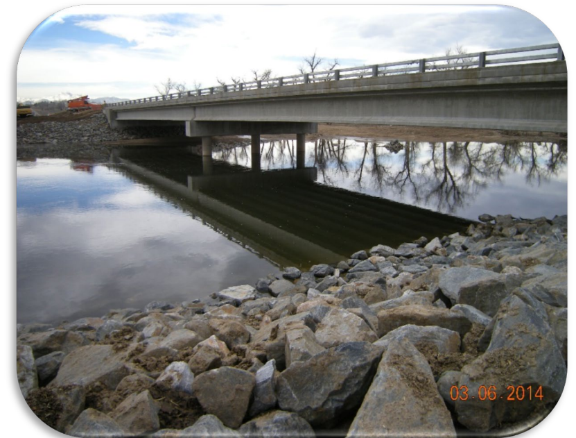
Region 4 SH 66 St. Vrain Bridge replaced in 2014
