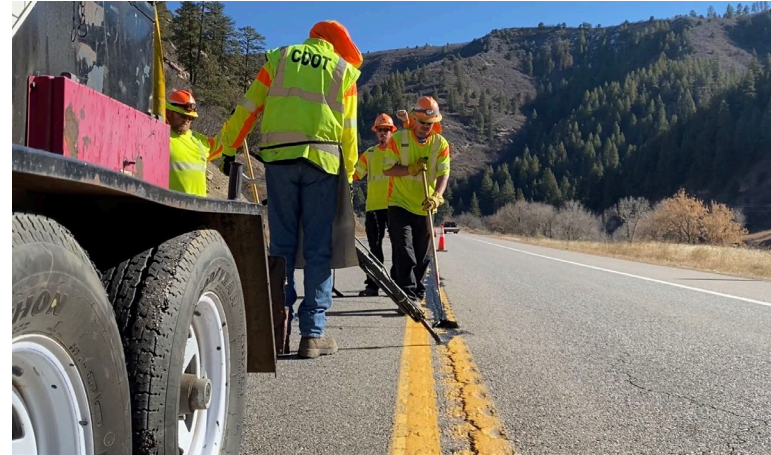
King Area patrols working along US 160 west of Durango
