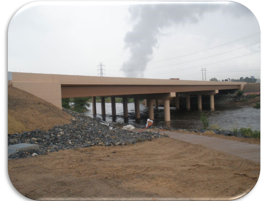
Region 1 I-76 over S.Platte replaced in 2016
